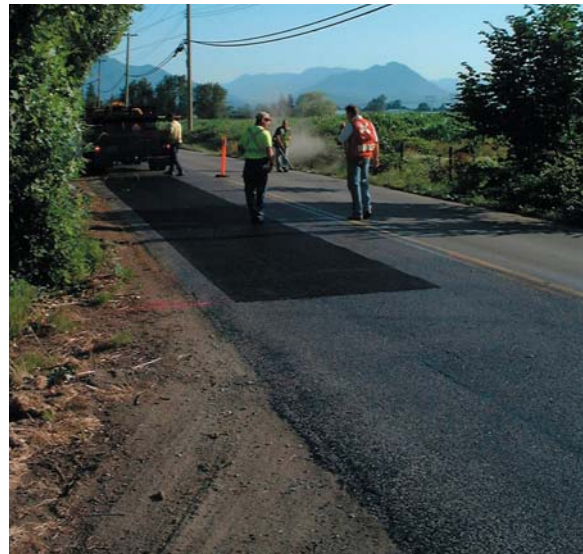
Placed RoadGrid in outer wheel wells
