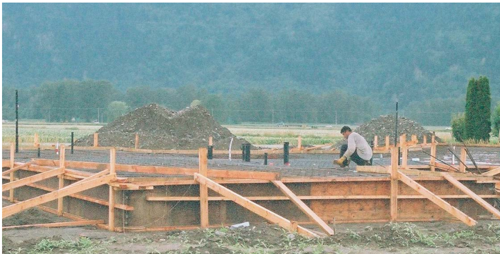
"Foundation being constructed over Checkmate's RigidGrid BX2525"
